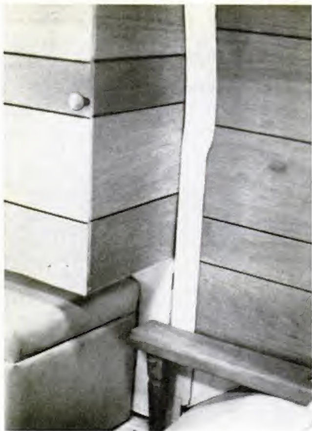
RIGHT MID-SIDE showing 2x4 runner which bed rests upon. At top left is door-mounted clothes closet. The portable chemical-toilet fits neatly below
